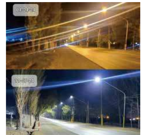
(Before/After):PENEL LED Street lights significantly improved the road lighting in San Juan province beside the Andes mountains in 2024 in Argentina
