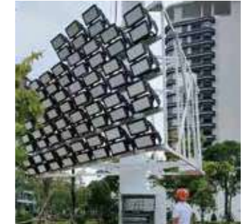
Football field installing PENEL 500W Sports lights in 2024 in China
