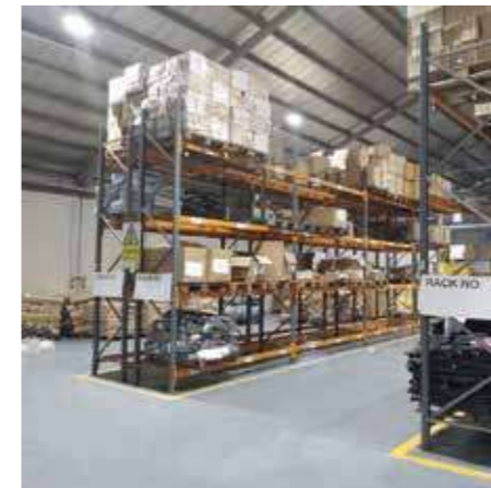
PENEL 200W LED High Bay lights were illuminating a warehouse in 2023 in Nigeria
